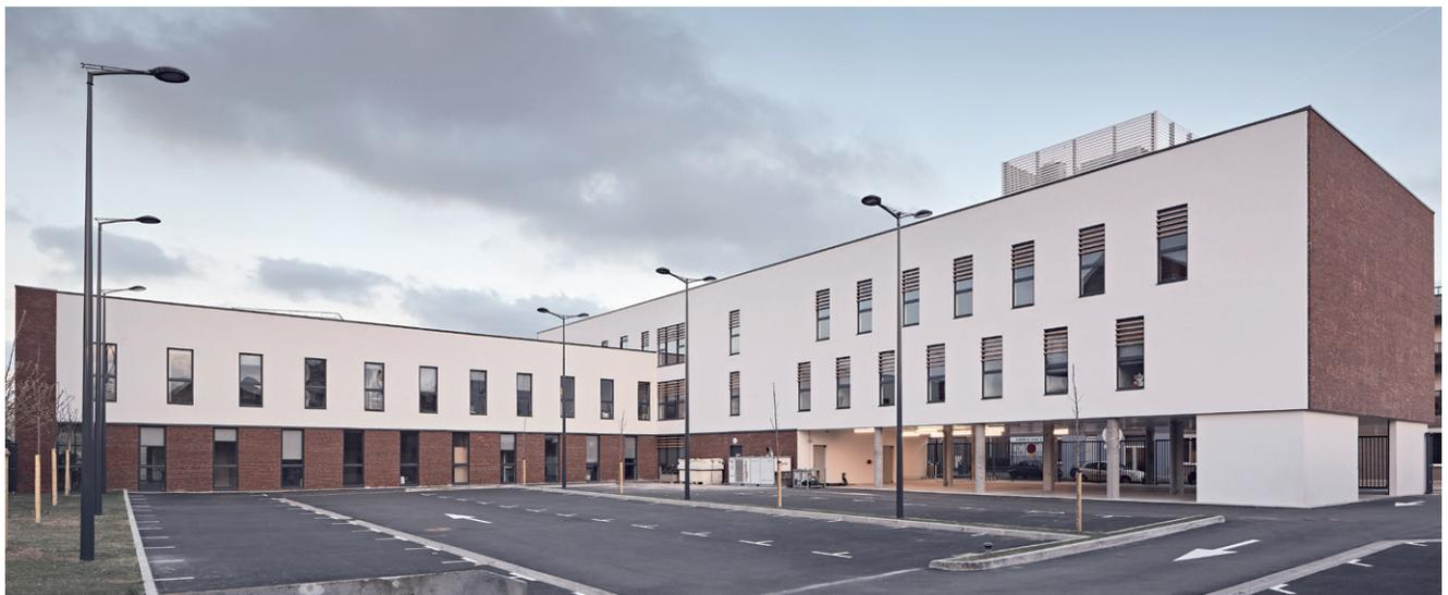
environmental approach : certified low-energy building High-performance building shell : external insulation, limited opening, brise-soleil, low-emissivity glass, green roof
